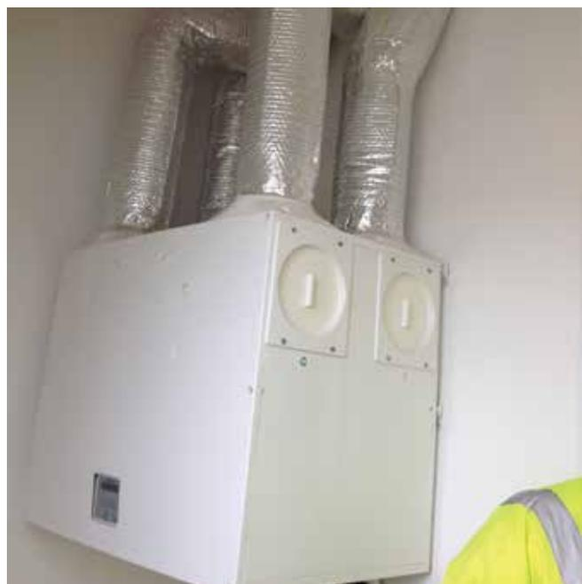
**Figure 9:** MVHR system installed in a Crest Nicholson home
