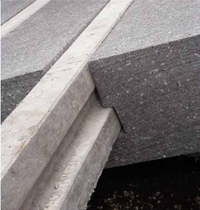
**Figure 7:** Floor insulation system used by Barratt Developments and Crest Nicholson (Courtesy of Springvale)
